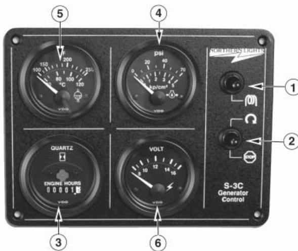
Figure 3-B: Series 3 Generator Control Panel
