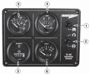
Figure 6-a: Series 3 Generator Control Panel
