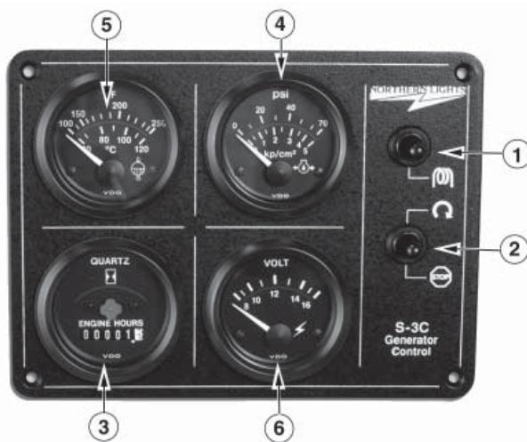
Figure 5: Series 3 Generator Control Panel
